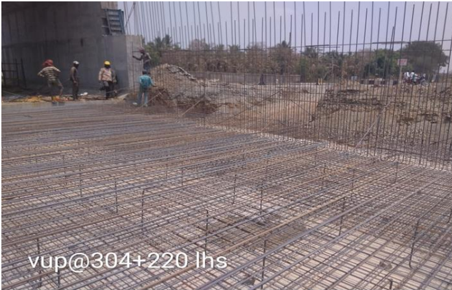
304+220 VUP Reinforcement in Progress
