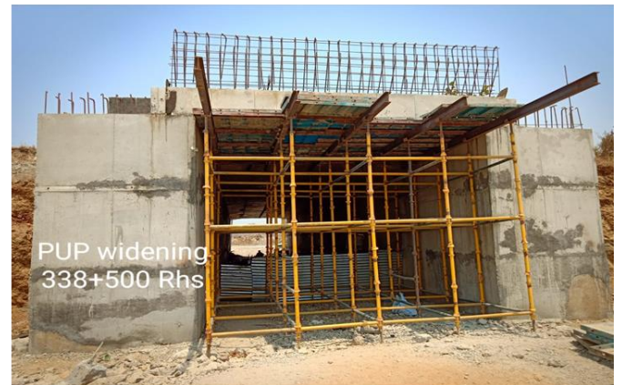
338+500Rhs PUP widening
