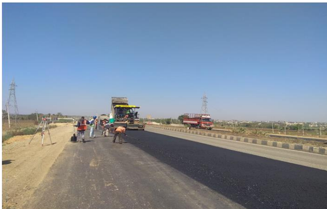
DBM Laying (Lane-2) at 329+500 LHS
