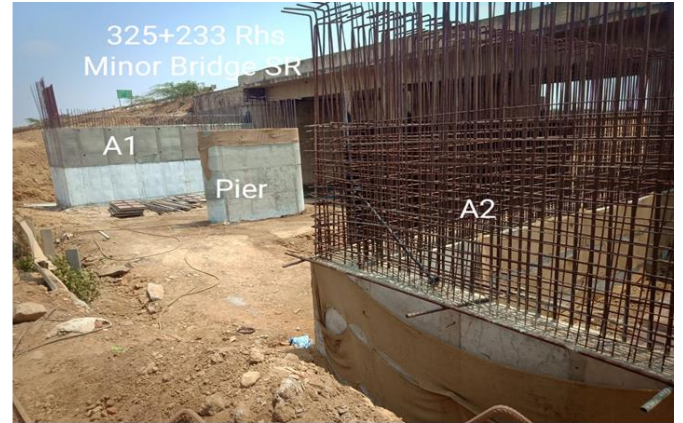
325+233 RHS Minor Bridge
