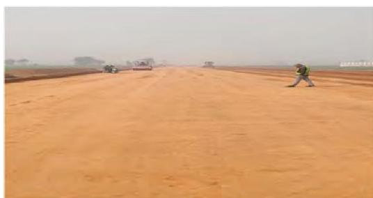
Subgrade 1<sup>st</sup> Layer Compaction in Progress at 25+500 Km
