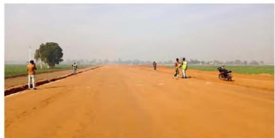
Subgrade Top Level checking in Progress 25+700
