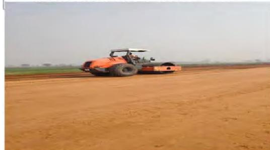
Subgrade Layer Compaction in Progress 25+600 km
