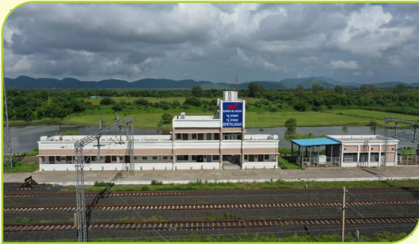
Dedicated Freight Corridor Project, CTP-12
