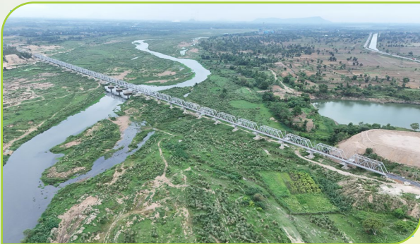
Open Web Girder Over Hasdeo River, CEWRL Project
