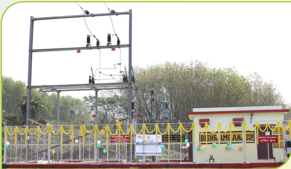
Bishramganj SSP, Railway Electrification Pkg 2
