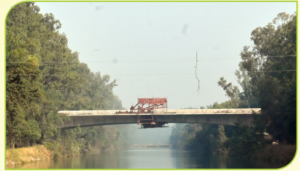
63m Balance Cantilever Span Ludhiana – Rupnagar Project
