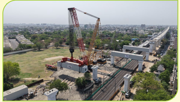
MAHSR C – 7 Project, Ahmedabad
