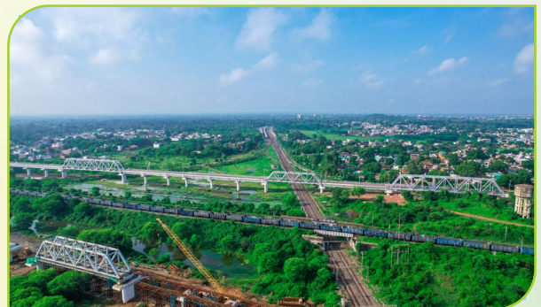
Katni Grade Separator Project
