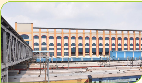
Backside View of Santragachi Station Building
