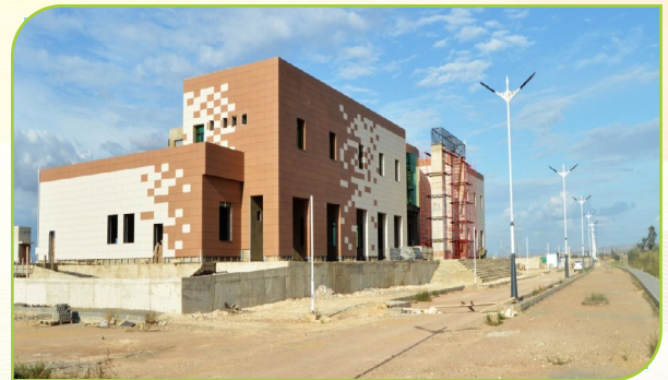
Relizane Railway Station, Algeria
