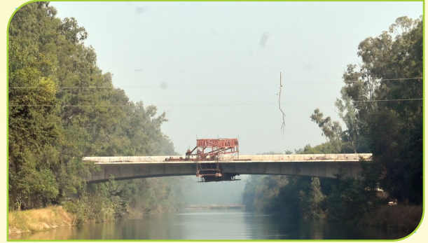
63m Balance Cantilever Span Ludhiana – Rupnagar Project
