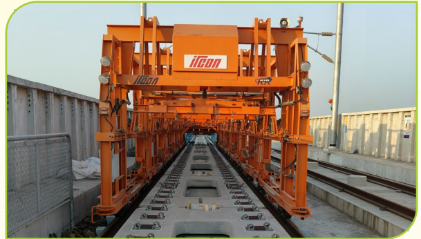
MAHSR T – 2 Project
