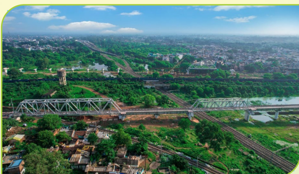
Katni Grade Separator Project
