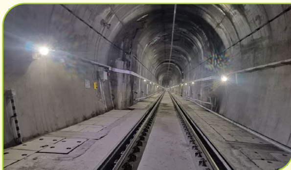
Tunnel T-52, D-Shape & Horse Shoe Shape, USBRL Project
