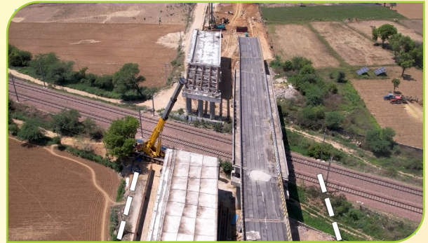
Gurgaon – Rewari Highway Project
