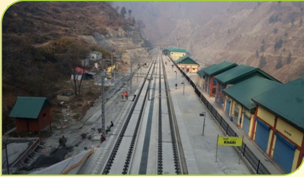
Khari Station Yard, USBRL Project, J&K
