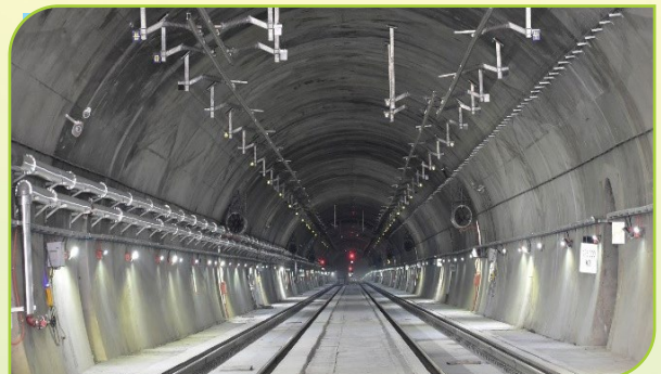
ROCS Erection in Tunnel T-50, USBRL Project
