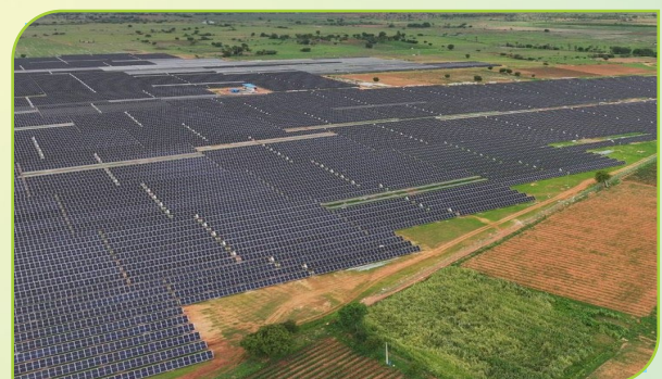
Solar Power Project of Ircn Renewable Power Limited
