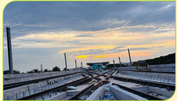
Scissor Cross Over with Track Centre 12 M, Chennai Metro Rail Project
