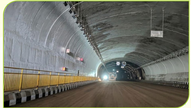
Bhoj Morbe Expressway Project
