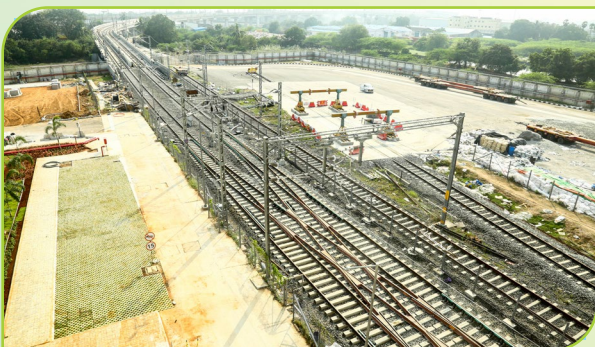
Poonamallee Depot, Chennai Metro Rail Project
