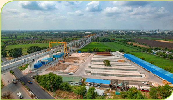
MAHSR T – 2 Project
