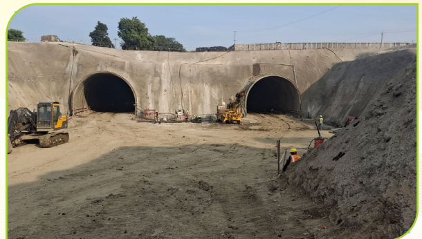
Indore Budni Tunnel T1 Project
