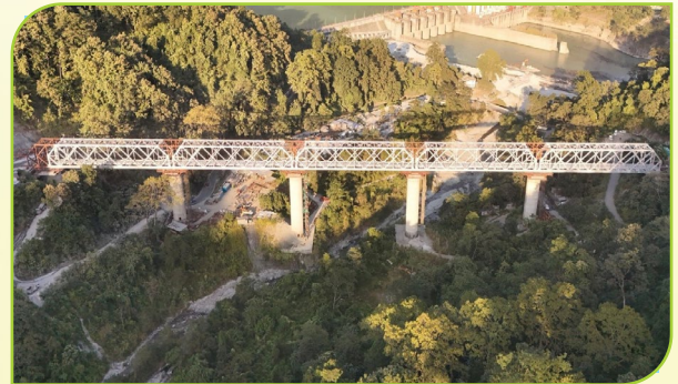
Bridge No. 3, Sivok Rangpo New Rail Line Project
