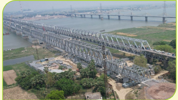
Rampur – Dumra Tal Rajendrapul Addl. Bridge & Doubling Project
